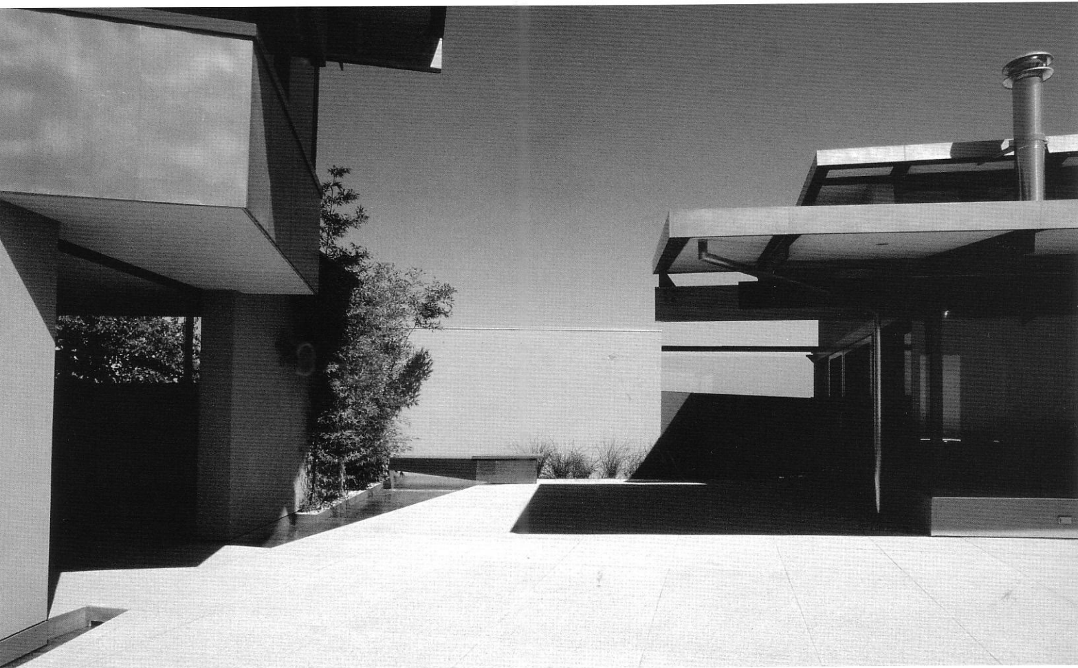
ABOVE: The void between the office pavilion, at left, and the screening room, at right, defines an outdoor room that extends into the paved courtyard. Continuing the tradition of the LA modernists, SMH designed the new residence for exterior as well as interior living.
